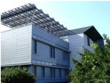
[The REC Conference Center](#) was refurbished in 2008 as a zero-emission building. Electricity is produced by solar cells, heating and cooling is based on heat pumps. Beside these passive elements (natural lights, shadowing) and efficient lighting system, minimized electricity consumption also help reach zero-emission. The energy balance of the building is being monitored, data are available at:
